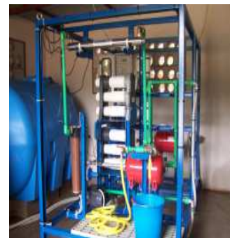
The filtration plant
